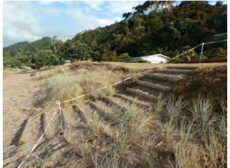
Three new sand ladders have been installed at Long Beach, Russell.
