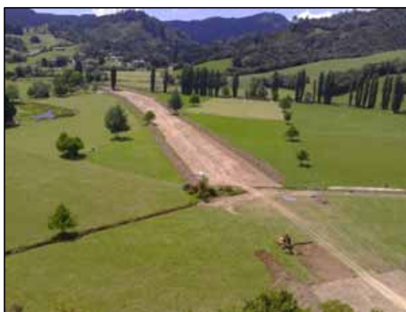
Kaeo River topsoil stripping for main stopbank
