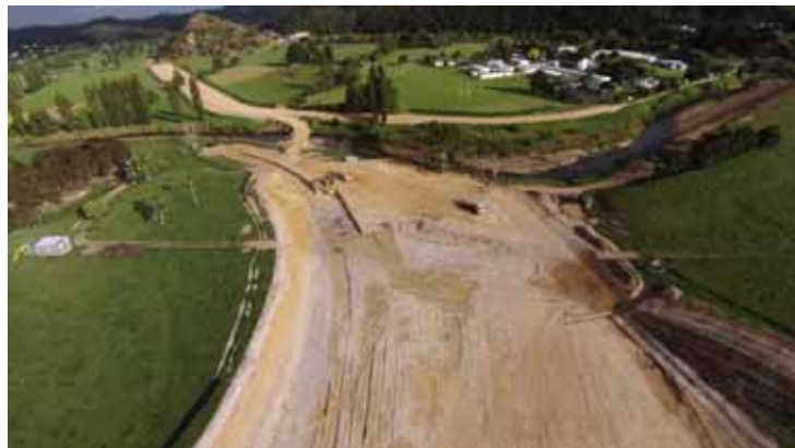
Kaeo River spillway, main stopbank and school stopbank/floodwall.
