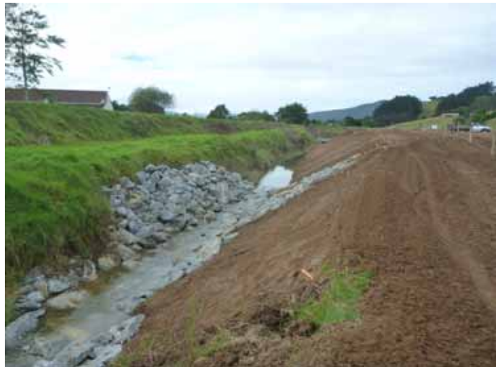
Grade Control on the Tarawhataroa Stream
