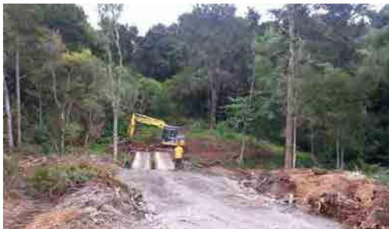
Kotuku Street Dam Utility Relocation – Temporary Stream Crossing
