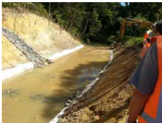
Stream Diversion – Inlet channel for the service spillway
