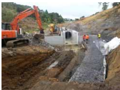
Inlet shaping and Gabion placement
