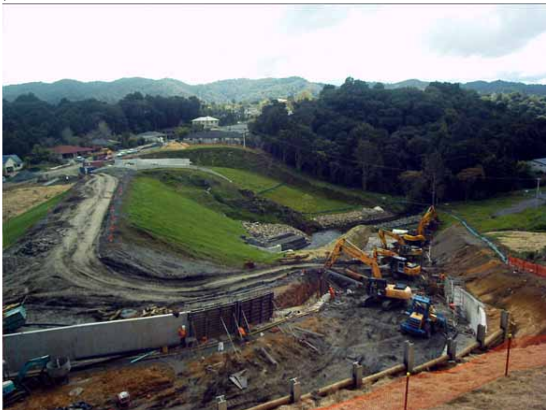
Kotuku dam 28 September 2015, work continuing on the right hand emergency spillway.
