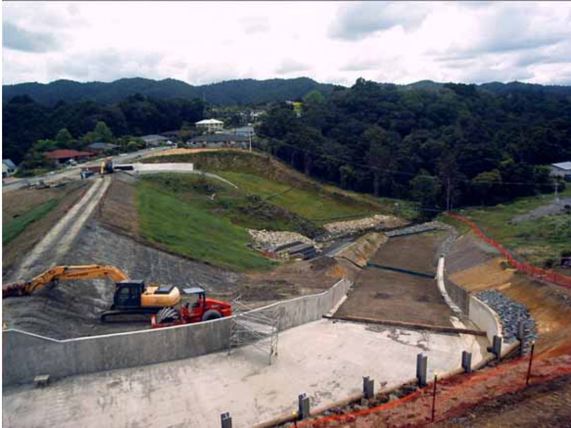
Kotuku dam 15 November 2015, final grading work continuing dam embankment.
