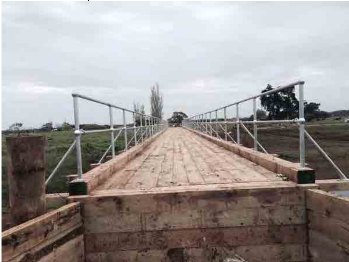
Matthew's Bridge nearing completion
