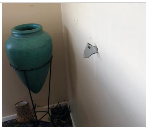
Glass imbedded in internal wall linings
