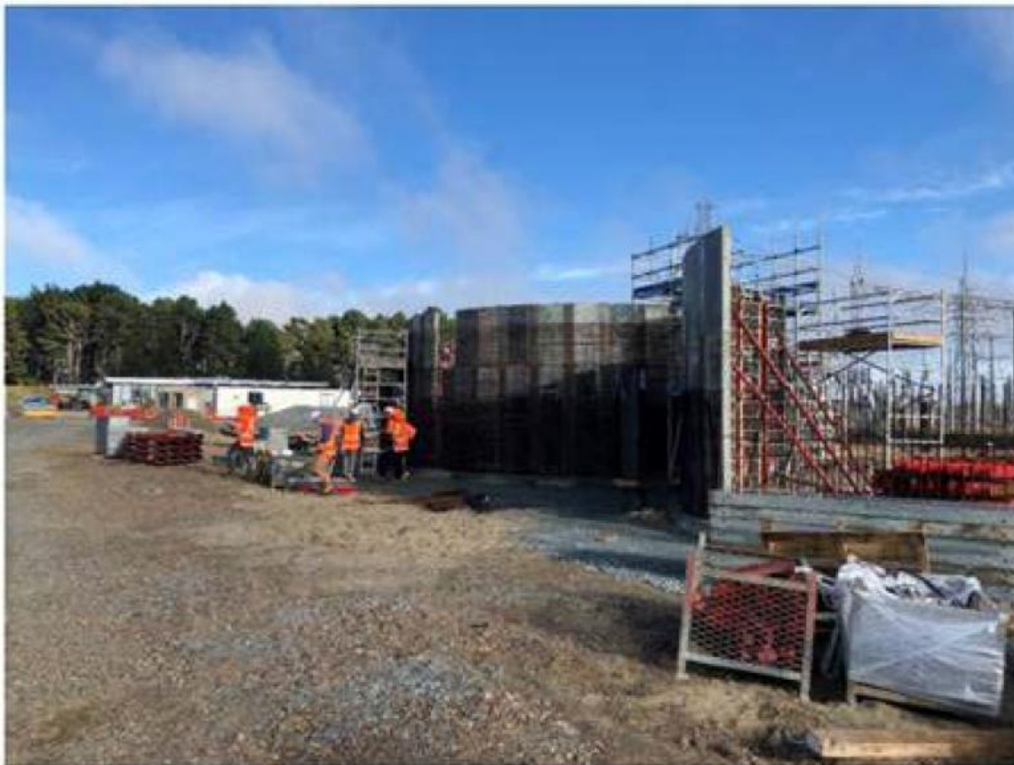
Wall formwork progressing for the first two fish tanks.
