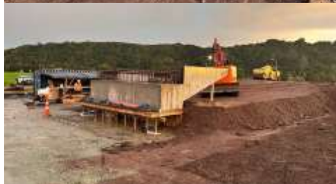
Abutment D concreted and backfilled
