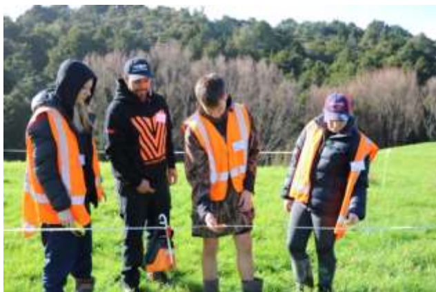
Temporary electric fencing – powering up, testing voltage and finding faults
