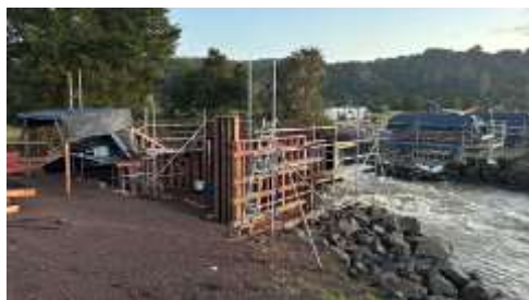
Abutment A looking East to Piers B and C
