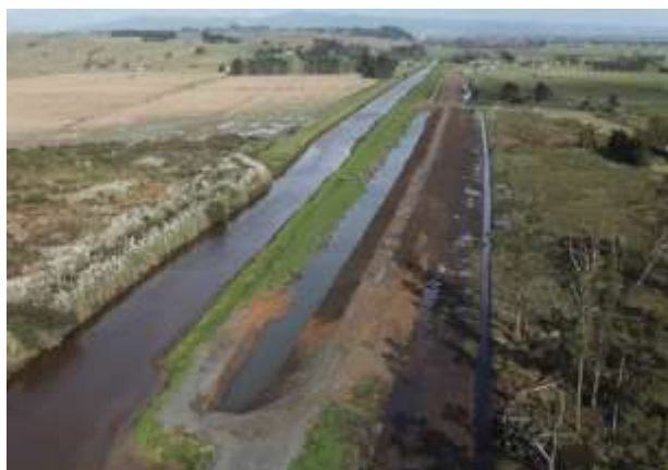
Lower Whangatane Spillway (35% complete) – Looking South.
