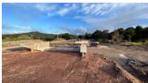
View looking West from Abutment D
