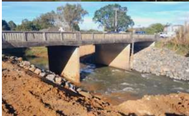
SH1/ Waikuruki Bridge (65% complete) – Looking South.
