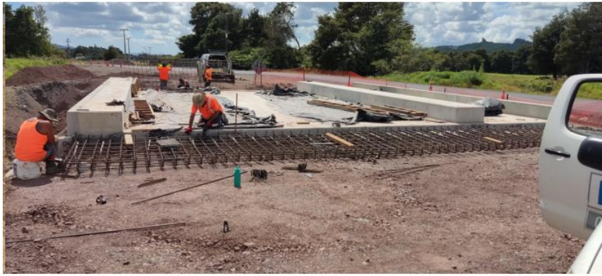
Photo 2. Barfoote steel fixing for settlement slab.
