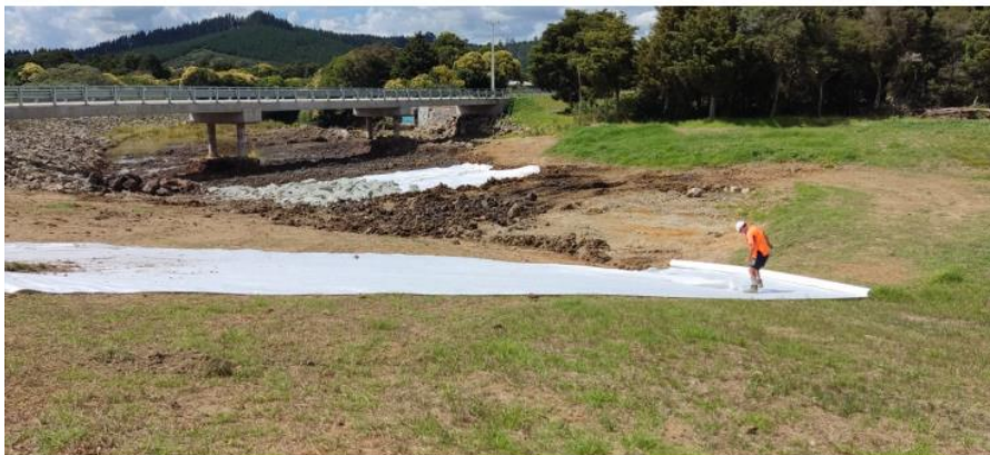
Photo 4. Geotextile being laid.
