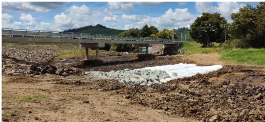
Photo 3. Excavation under bridge and downstream with lime rock placed.
