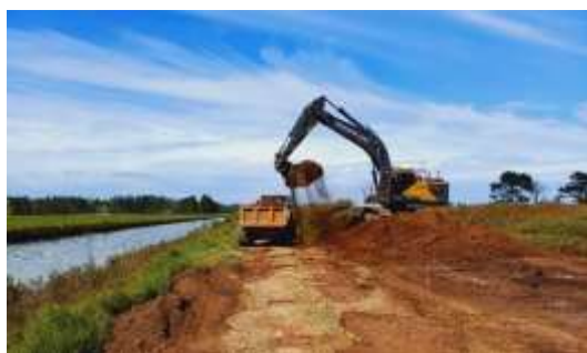
Excavation of Old Stopbank
