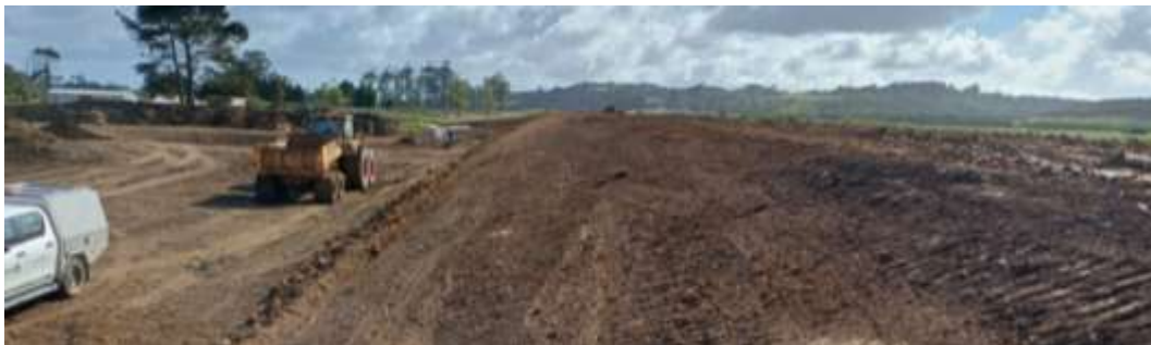
Newly formed stopbank looking North.
