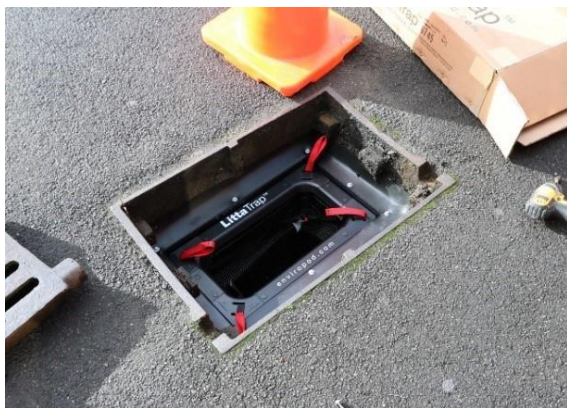
Litter trap being installed at the council's Water Street office carpark
