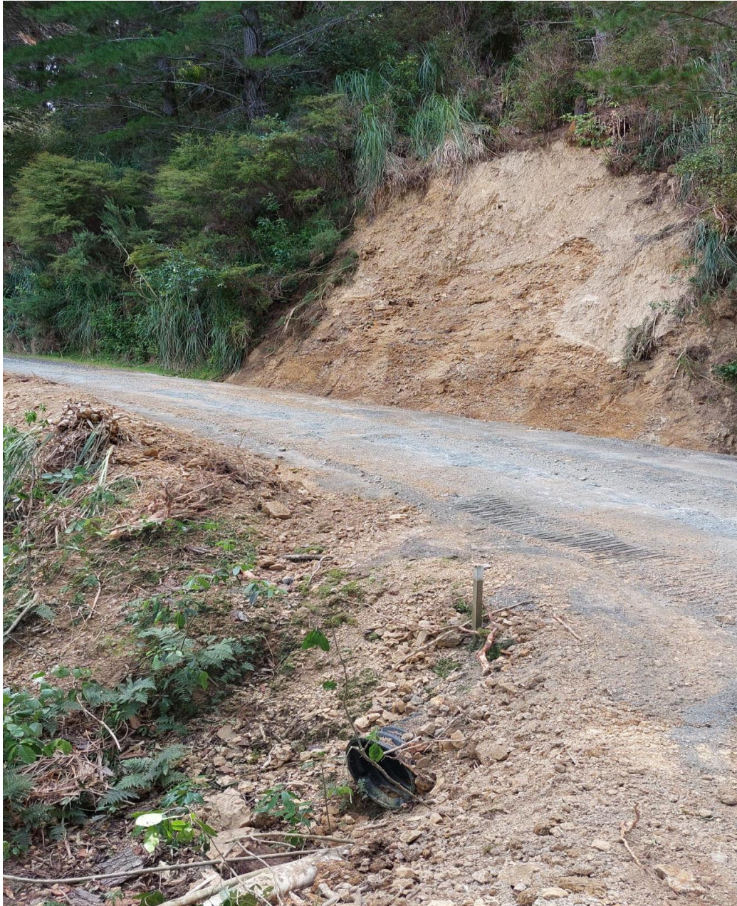
Tree removed and slip material cleared Dec 2021
