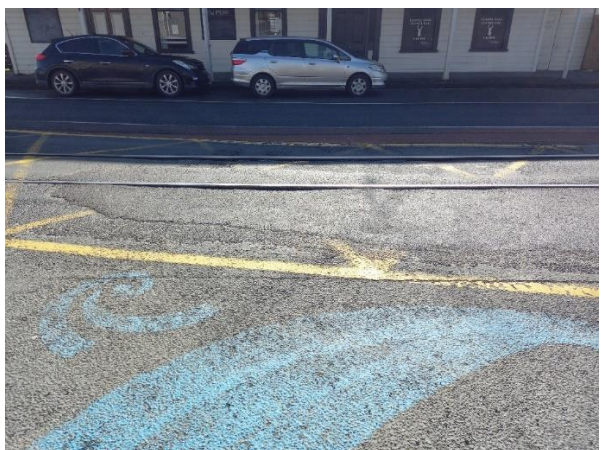
Kawakawa rail crossing – AFTER TEMPORARY REPAIR by Waka Kotahi
