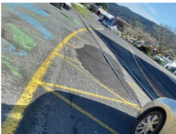
Kawakawa rail crossing – AFTER TEMPORARY REPAIR by Waka Kotahi
