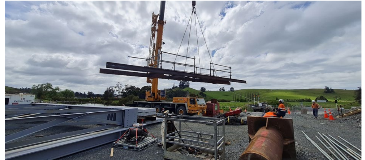
(Image: Craning the temporary staging into place at Otaika Creek)
