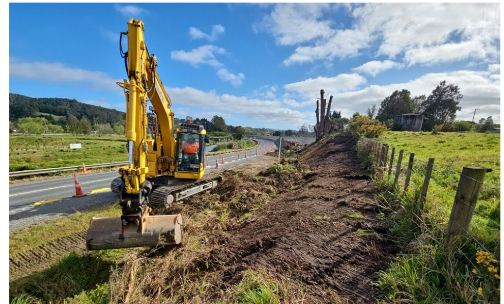
(Image: Starting work at the southern tie-in)
