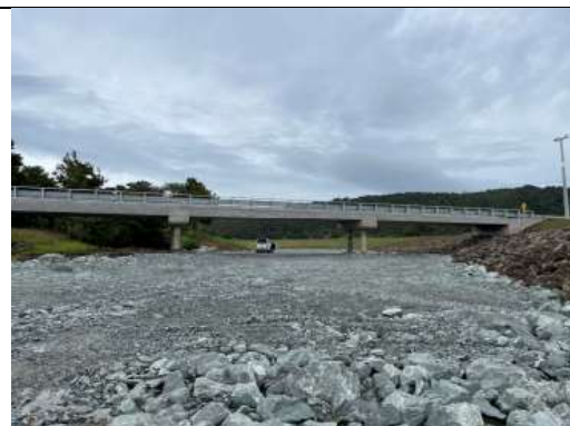
Spillway transition under Pokapu Bridge (downstream looking up)
