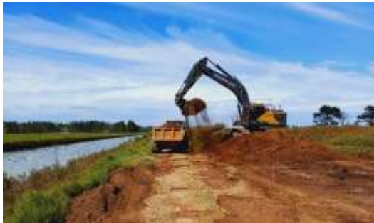
Excavation of Old Stopbank
