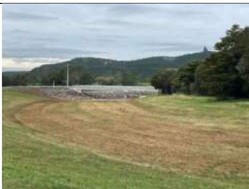
Spillway transition under Pokapu Bridge (upstream looking down)
