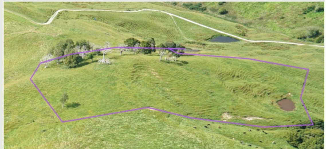
Oblique photography of Area 1, demonstrating areas of slips and scars from previous erosion
