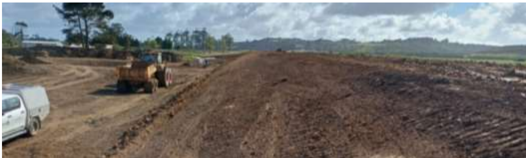
Newly formed stopbank looking North.
