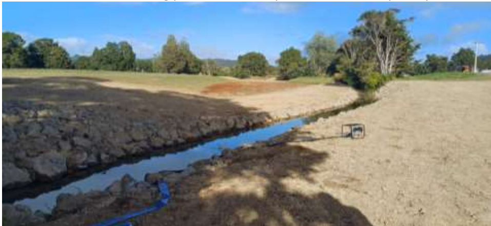
Otiria Spillway transition through creek
