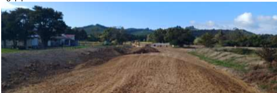
Final portion of the stop bank construction
