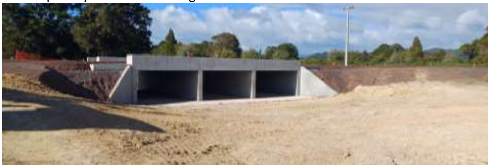
Ngapipito Road Box Culverts
