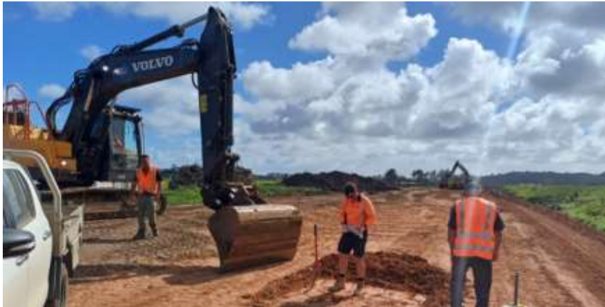
Nuclear Density testing underway.
