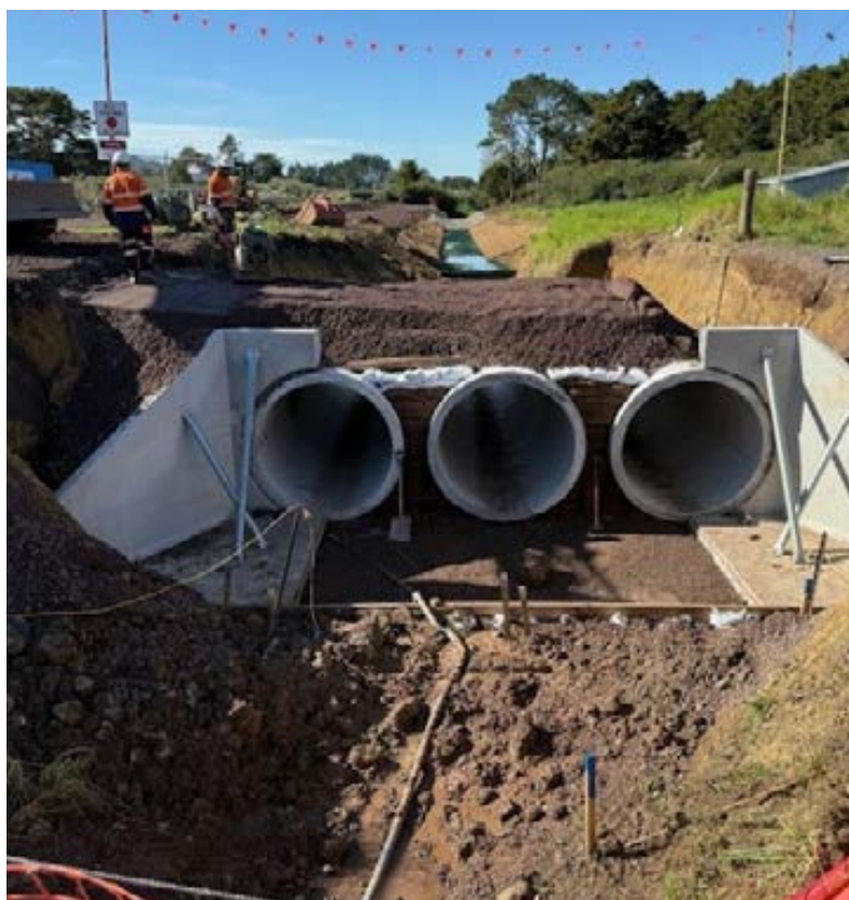
One of the culverts being installed at Otiria rail yard.
