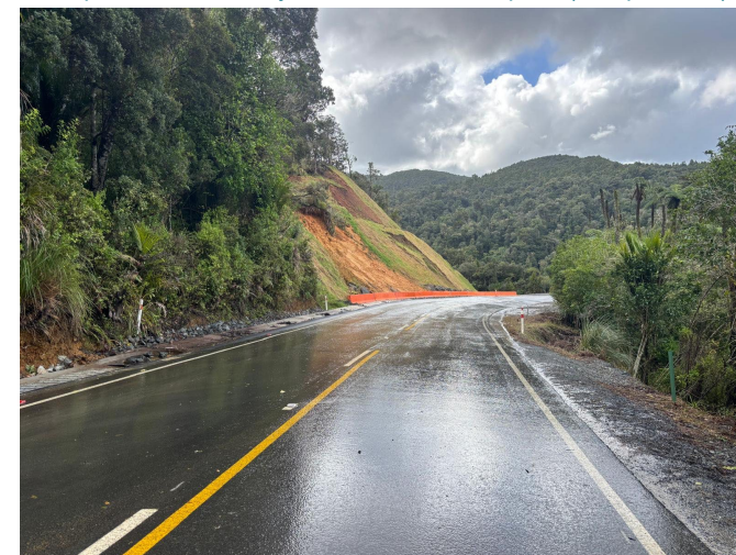
Slip at site A11 cleared & concrete barriers in place (2 May 2025)
