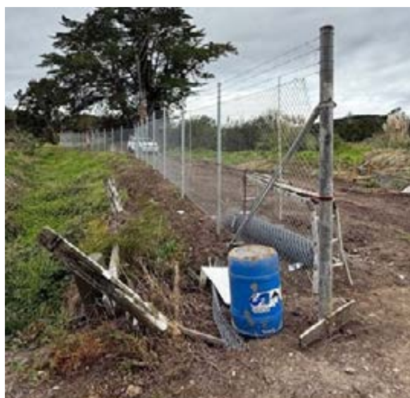
Mesh security fencing installed along Otiria Road.
