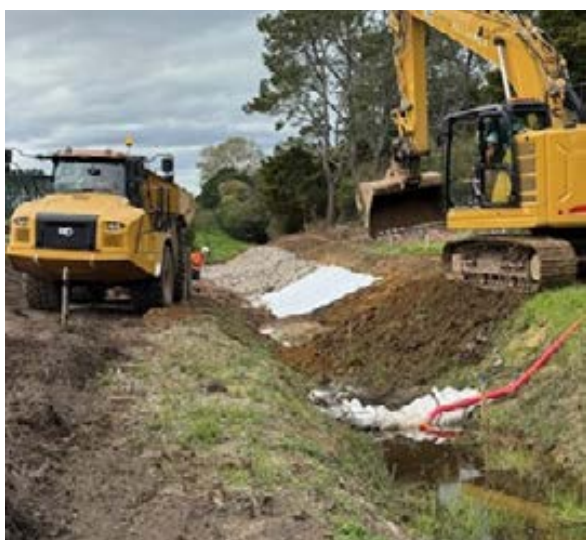
A swale channel being dug out and lined, before a layer of stones (known as Rip Rap) are added.
