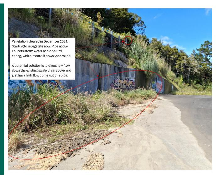
Undermined headwall at Woods Rd Floodwall
