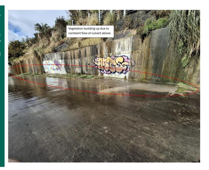
Excess water increases vegetation in the rest of the spillway.
