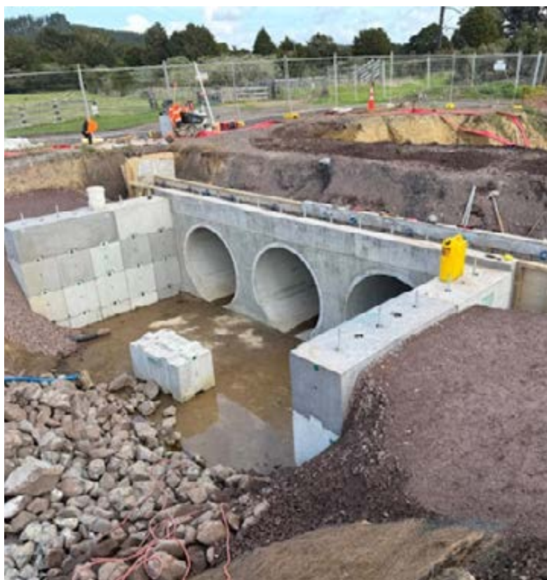
One of the barrel culverts being built
