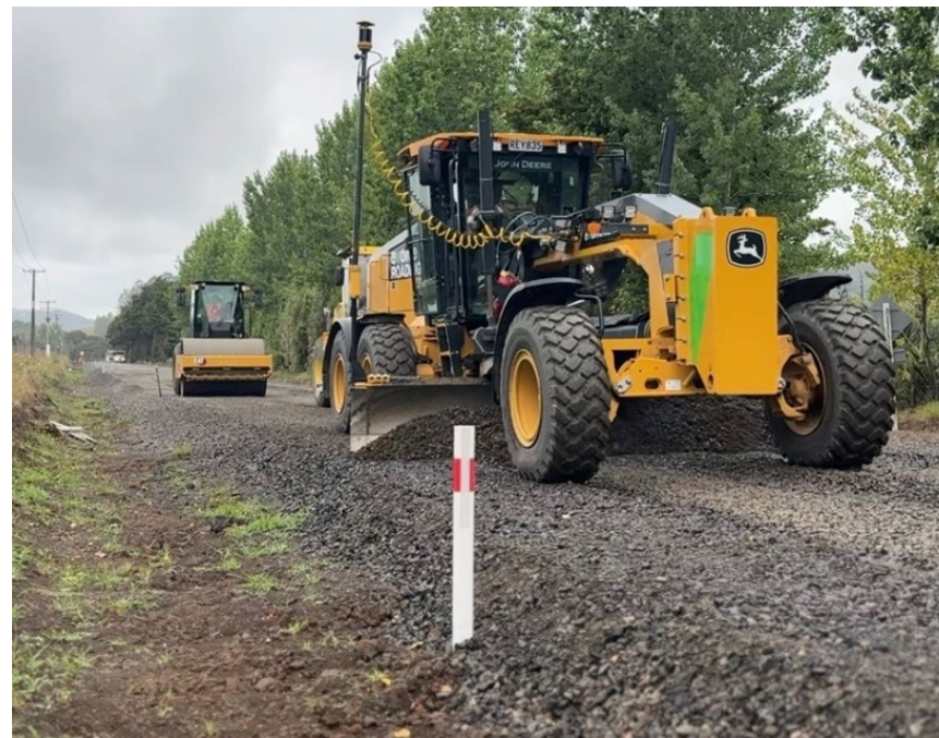
SH10 Oromahoe road rebuild in progress, pictured is the overlay being installed (January 2026)
